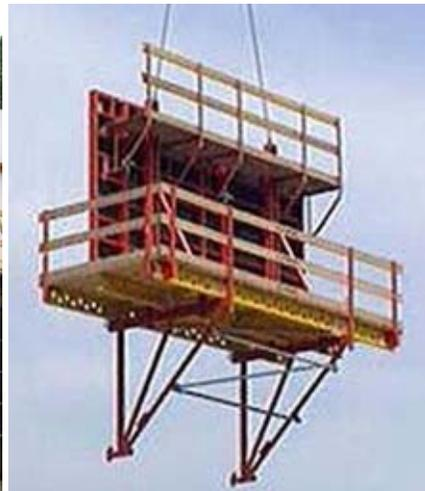
**Figure 7:** Movement to next lift via crane
