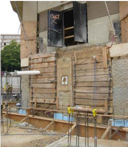
**Figure 13:** Underpinning - interpier beam/wale system (Fichandler)
