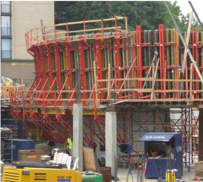
**Figure 8:** PERI RUNDFLEX formwork prepared for a lift pour
