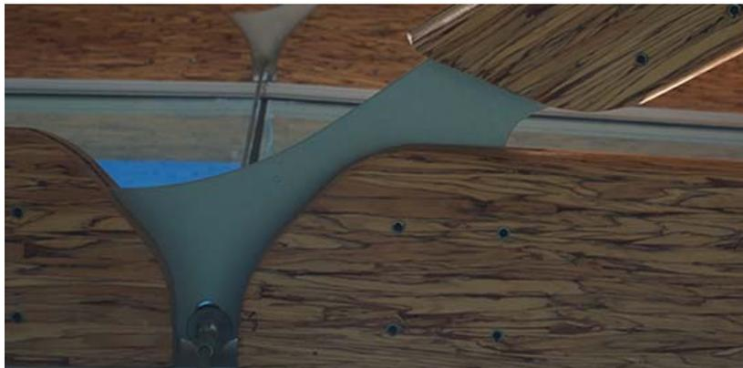
**Figure 12:** This detail shows the connection of the support arm and muntins to the aluminum plate with (4) tight-fit pins. Also shown is the intersection of the support cable with the aluminum plate.
