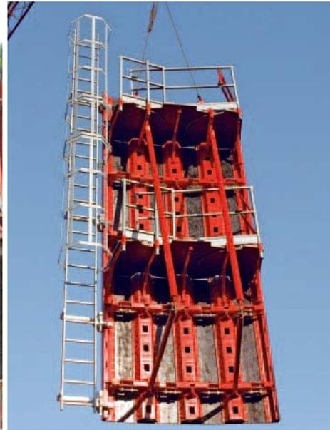
**Figure 9:** Movement to next lift via crane
